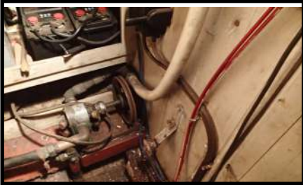
Pumpe montert i maskinrom
